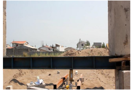
Fig.1. A view of pile load test
