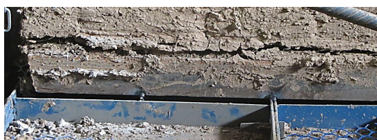
Figure 3: The failure of wall under lateral load
